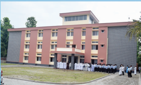
Mariam Niwas (Sisters's Hostel) at Nagaon
